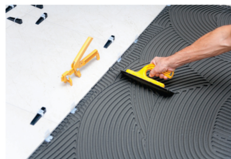
Stap4 : Apply adhesive & fix tiles
